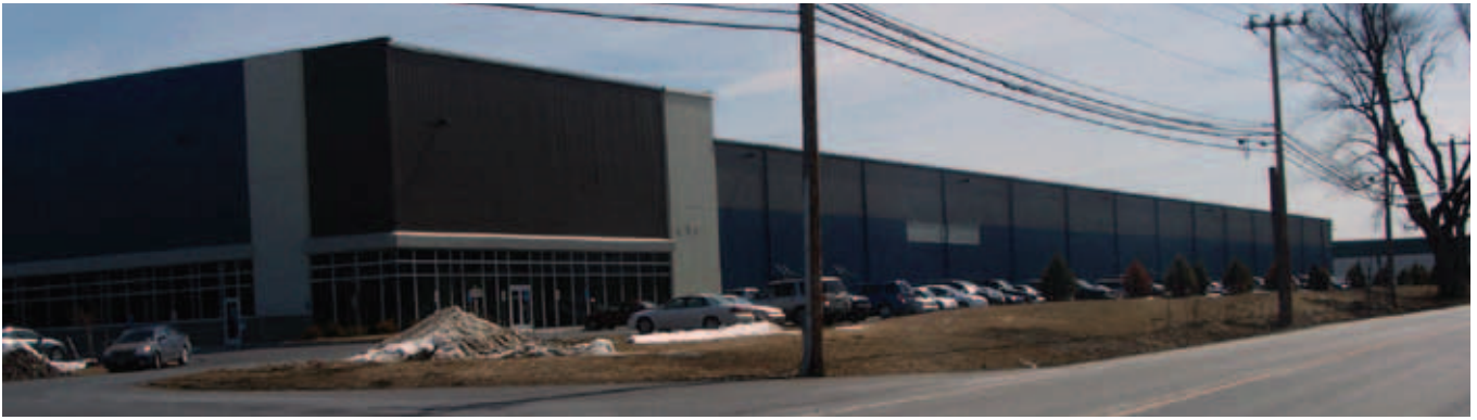
Communications Test Design, Inc. in the Glenville Business & Technology Park
